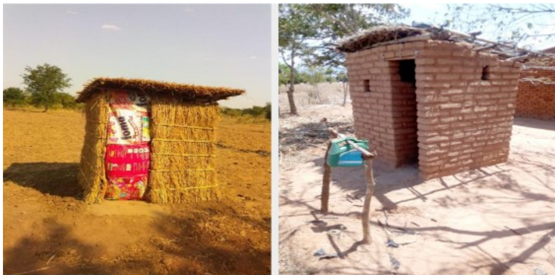
Figure 22: Nature of pit latrines in Rumphi Water and Sanitation Services Improvement Project area: one type made with grass material and no hand washing facility (Left) and another type constructed with bricks having a hand washing facility outside (R)
