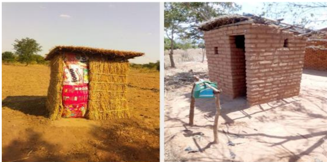
Figure 26: Nature of pit latrines in the Rumphi Water Supply and Sanitation Services Improvement Project area: one type made with grass material and no hand washing facility (Left) and another type constructed with bricks having a hand washing facility outside (R)
